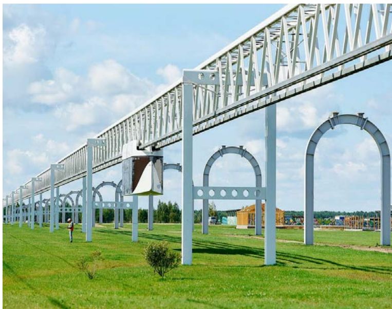
Fig. 4 – SkyWay track structure of rigid type (rail-string truss for movement of both suspended and mounted rolling stock) – Maryina Goroka, 2019
